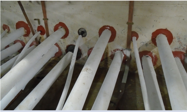
Entry point with test installation of 2 seals
