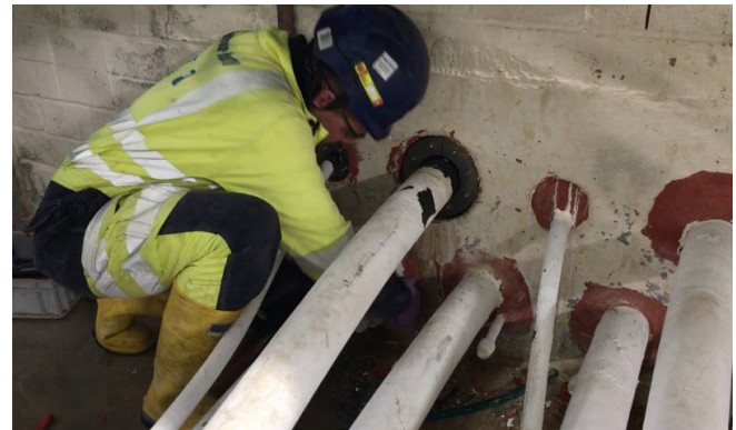
Installation of HRD 188-1G-1/97
