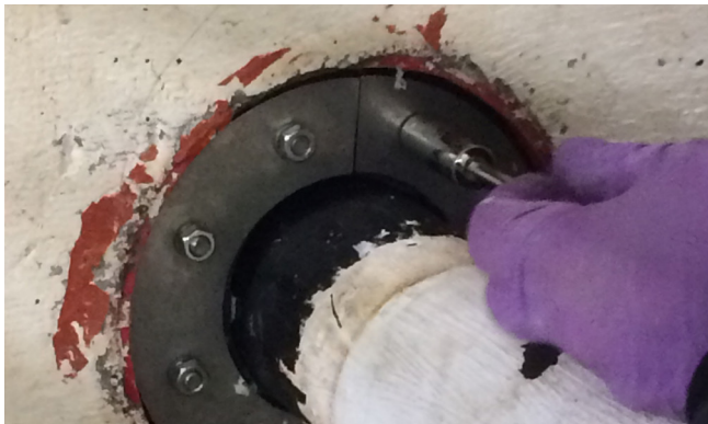
Installation of HRD 188-1G-1/97
