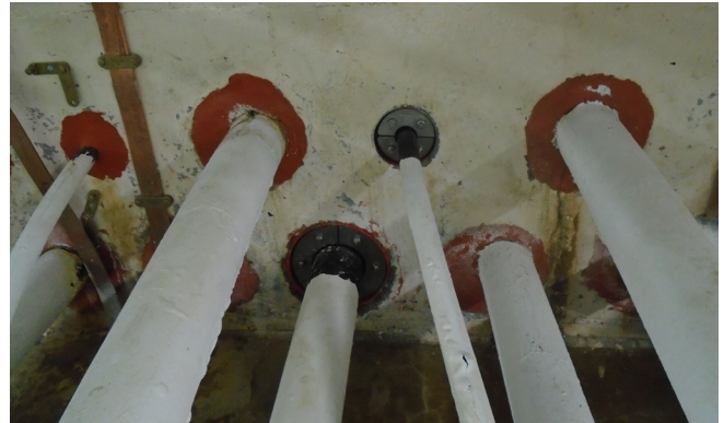
Test installation of 2 seals
