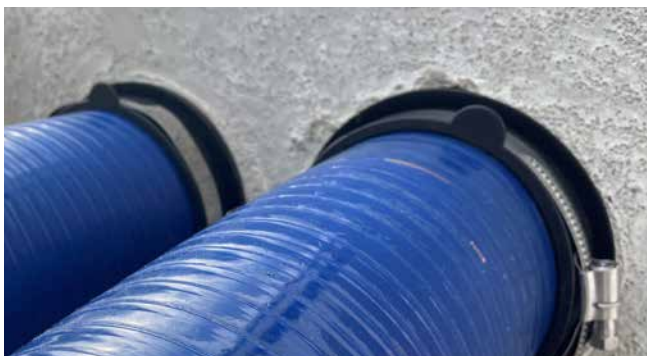
HSI150 KMA instalado
