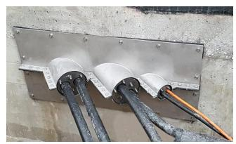
Solution: Overmeasure of a protrusion flange in split-design with different pipe socket outlets in relation to the exit angle of the cable. Image: Cable entry into the service duct
