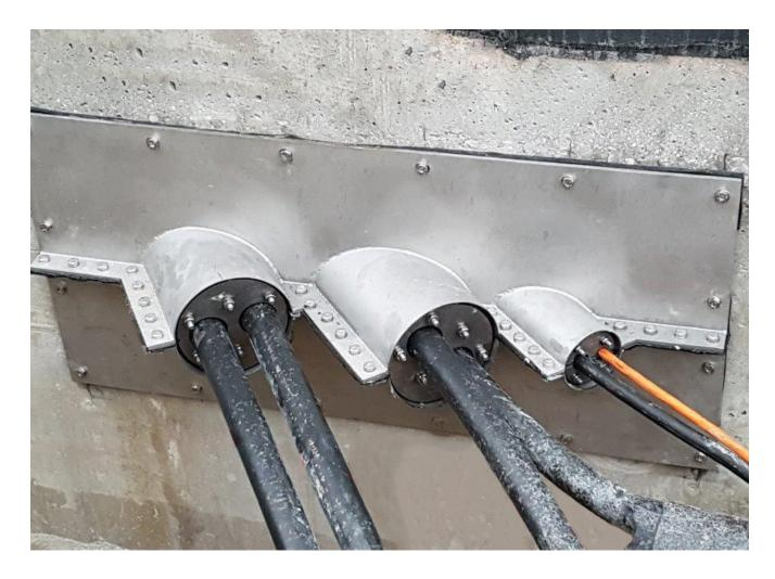
CABLE ENTRY WITH STAINLESS STEEL FLANGE HRD2X150-1X80
