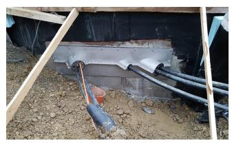
Image: Cable outlet on the service duct
