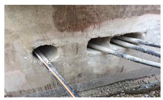
Special feature: Cables enter in and out of the service duct at varying angles. The position of the cables can not be altered. Image: Cable outlet on the service duct
