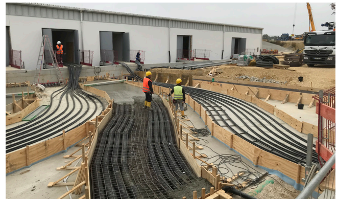
Concreting the duct connection between the new construction and existing buildings.
