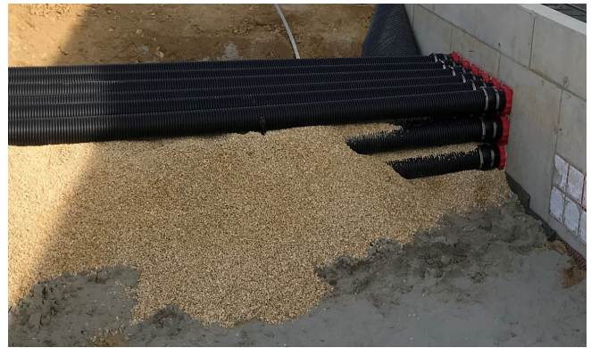
Fully installed duct to HSI 150 wall insert
