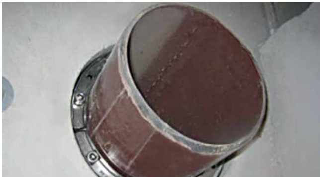
HSD200 1x160 b40 A2/EPDM55 – drainage SML pipe
