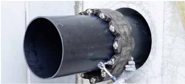
GKD400 – tightening of segments
