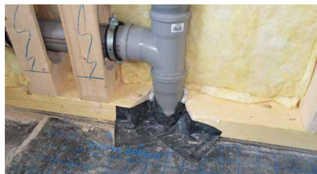
difficulty: integration of vapour barrier foil
