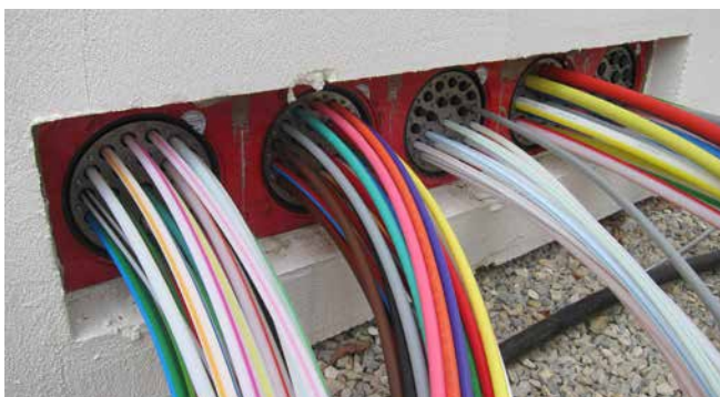
HSI150 wall insert fitted with HRD150 21x14 b60 A2/EPDM55 to seal micro pipes
