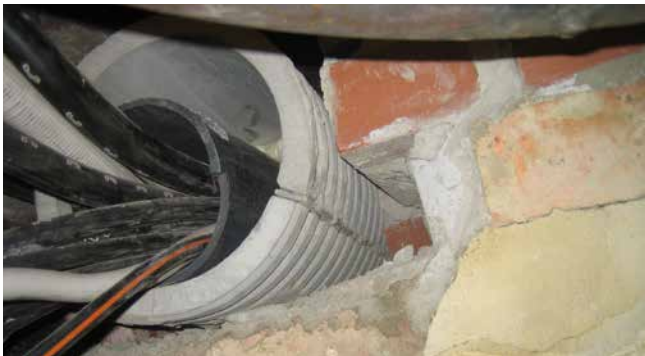
FZRG150/350 – refurbishment in masonry
