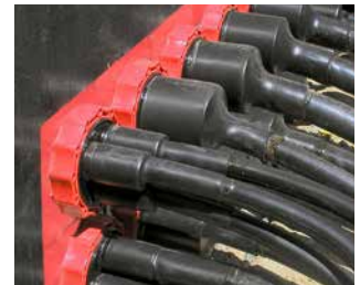
station entry: low-voltage cable sealed HSI90 D1x75 WS and HSI90 D3x32 WS
