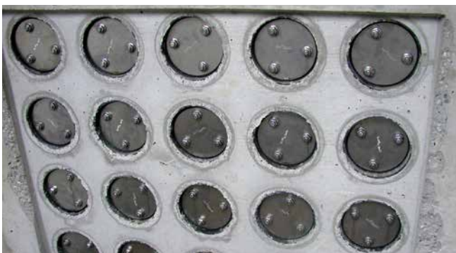
FZR100/240 – pipe section sealing
