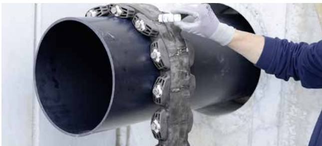
GKD400 – installation preparation with lubricant GM
