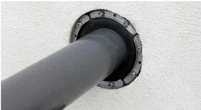
HSD200 1x159 b20 A2/EPDM55 "shaft seal"
